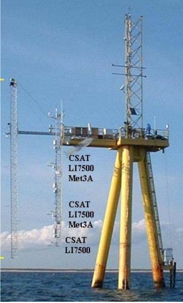
Figure 2: ASI Tower with the instruments mast.
