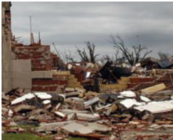
Figure 8: Damage to southwest wall to Greensburg High School. (Larry Ruthi, 2007)
