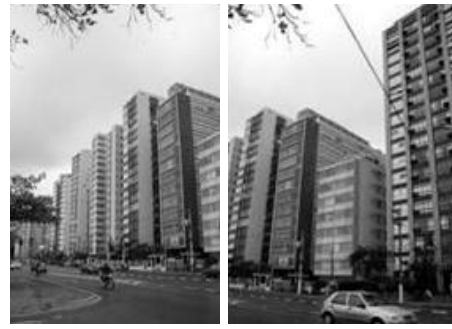
Figure 2: Buildings in the study area
