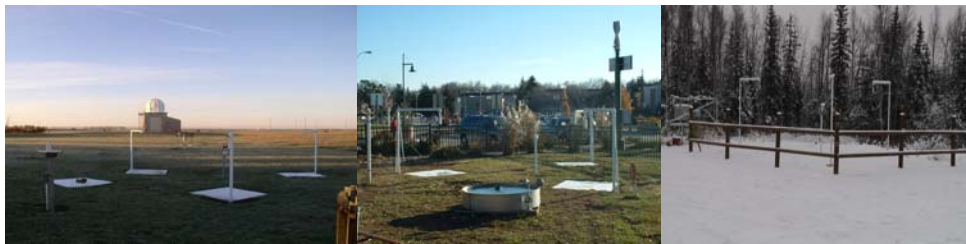
Figure 2: Site photos of complete installation from left to right: ABR, FCL and FAI
