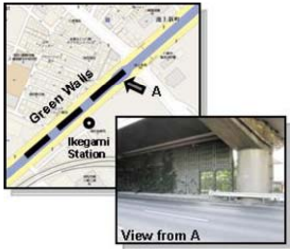
Figure 13 Green Walls Installed on the Industrial Road Divided into three parts, steel panels are installed on the center line of the Industrial Road between the ground level and the bottom of the elevated road.
