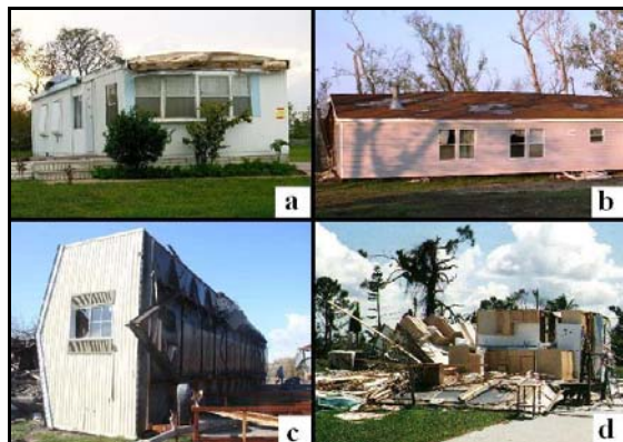
Figure 5. Various DODs to manufactured homes: a) loss of the roof covering (DOD 2), b) sliding of unit off its piers (DOD 3), c) rolling of home (DOD 5), and destruction of roof and walls leaving the floor in place (DOD 6).
