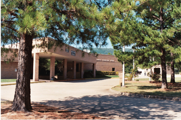
Figure 12. Kiamichi Technology Center at Talihina, Oklahoma.
