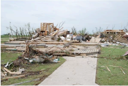
Figure 3. Remnants of House #2.
