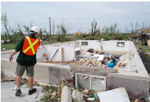
Figure 4. Foundation of House #3.
