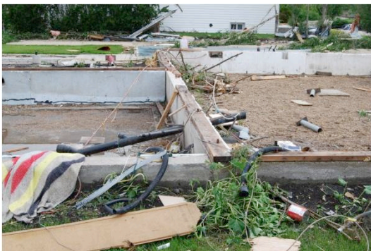
Figure 1. Foundation of House #1.
