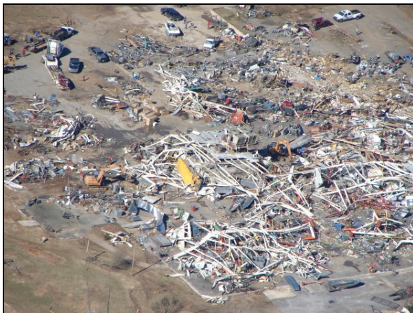
Figure 14: A boat factory was leveled at Clinton (Van Buren County).
