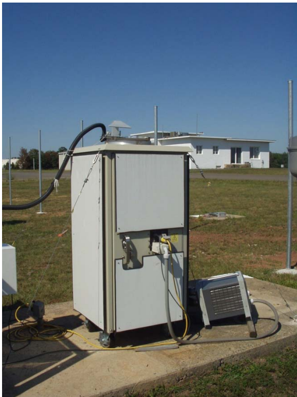
Figure 3. Micropulse Lidar with blower and air conditioner
