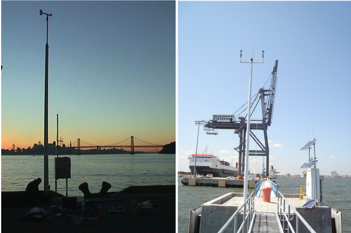
Figure 1. Left: Oakland Middle Harbor, CA wind-only station, with the San Francisco-Oakland Bay Bridge in the background. Right: West Pier, Port of Gulfport, MS is a standard PORTS water level station containing a full suite of meteorological sensors, complete with dual anemometers.
