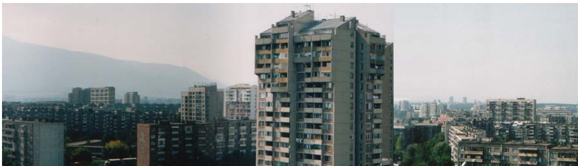
Figure 8. View from 40 m level of the Meteorological tower towards West
