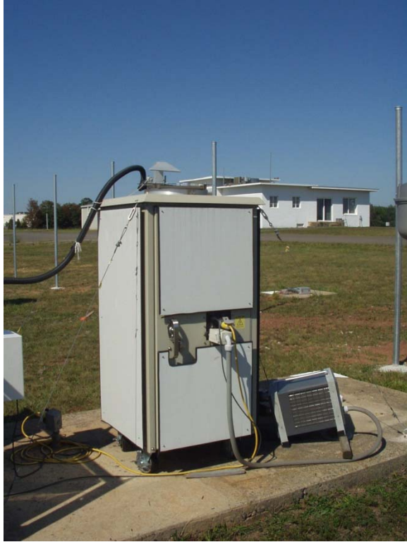
Figure 4. MicroPulse Lidar with blower and air conditioner
