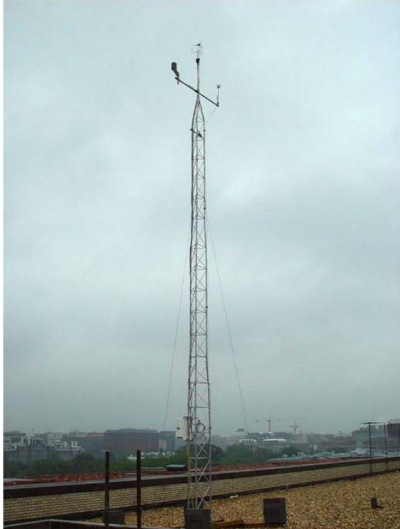
Figure 2. An example of a DCNet tower, showing a sonic anemometer at the top of a roof-mounted 10 m tower, with a standard meteorological instrumentation set mounted slightly below.
