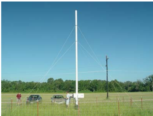
Figure 5.1 LDAR sensor at the Williams Airport in far north Houston
