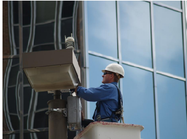
Figure 2. An OKCNET technician installs a traffic signal station.
