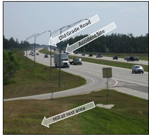
Fig. 9 Looking northeast from the rest area towards the accident site.
