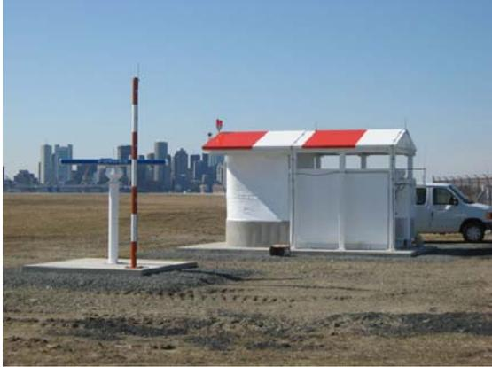
Fig. 2. Photograph of the W-Band Radar Shelter at Logan International Airport, showing the Boston skyline. The antenna (see Fig. 4) is housed in the cylindrically-shaped radome on the left.
