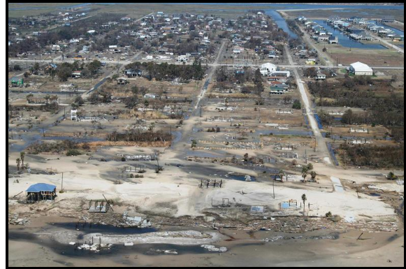
Figure 4. Wave action destroyed buildings near the beach (bottom of image) whereas buildings farther inland (top of image) remained intact.
