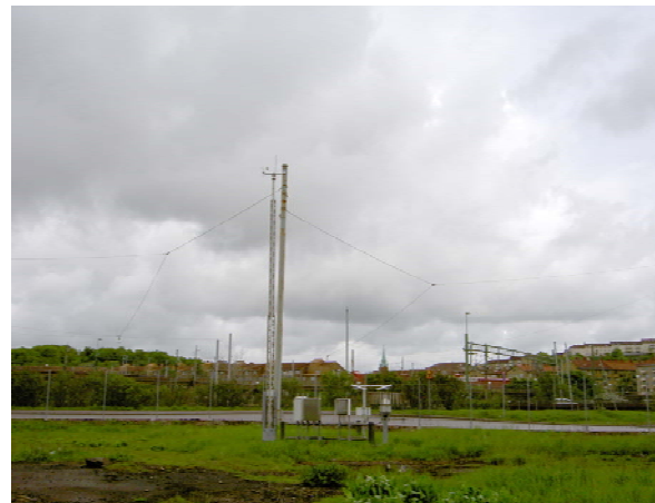
Figure 1. Gothenburg canyon site (top) and SMHI weather station (bottom).
