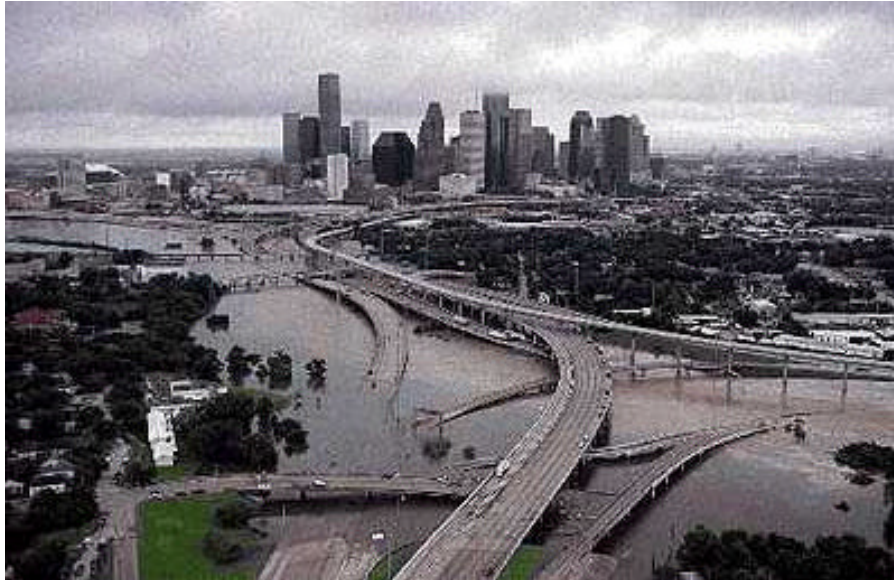
Figure 1. The Interstate 45/Interstate 10 interchange north of downtown Houston on Saturday, 9 June 2001, after Tropical Storm Allison. [Courtesy of DallasNews.com.]
