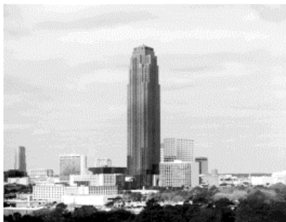
Figure 1. Williams Tower, looking to the southwest. Observations were taken from the top parapet.
