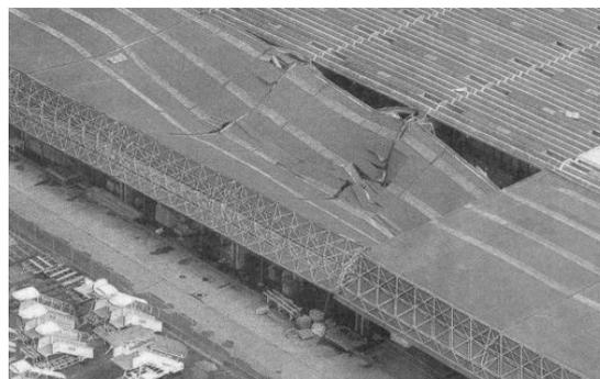
**Figure 5:** Aerial view of the damage caused to the SPIA cargo terminal in the 2 April 1999 thunderstorm event.
