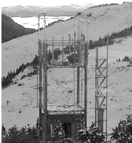
Fig. 1. Photograph of the Eagle Crest equipment tower.
