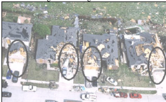
Figure 6. Garage failures (circled) on homes that faced the wind.
