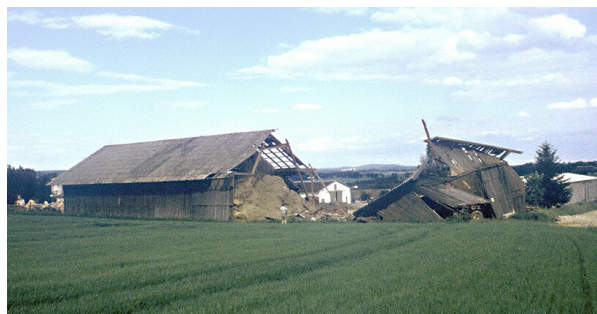
Figure 1. A barn, partially damaged by one of the May 31, 2001 tornadoes in Mrzkovice (central Czech Republic).
