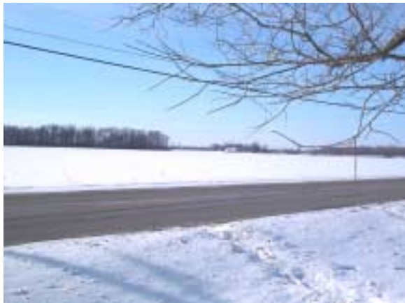
Figure 12. Ohio road test section
