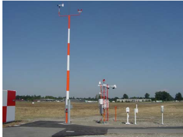
Fig. 3. Installation showing Primary Group.
