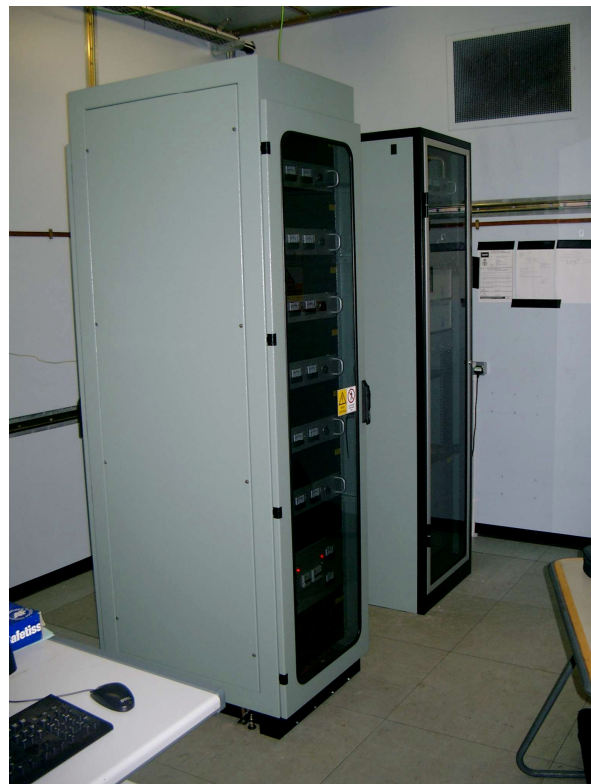
Fig. 3 LHS rack mounted transmitters, RHS two electronics cabinets house the basic hardware
