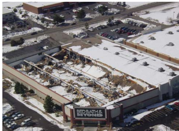
Figure 4. Bed Bath & Beyond collapsed roof from March 17-19th snowstorm. Photo taken by John Fischbach, City of Fort Collins.
