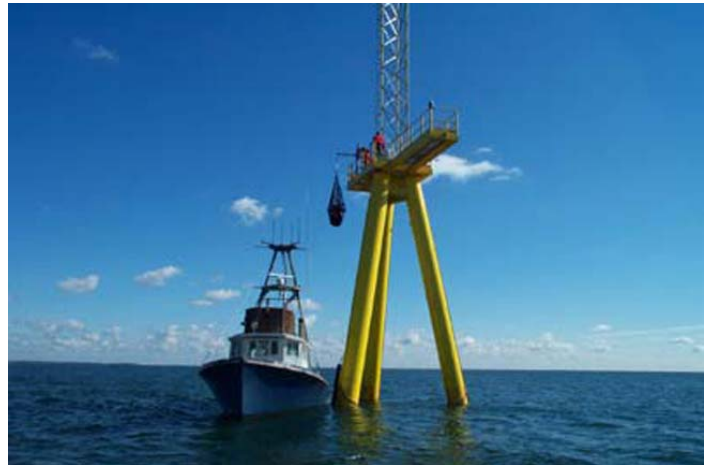
Figure 2. Photograph of the air-sea interaction tower, constructed as part of the CBLAST-low program. The tower is at a water depth of 15 m. The deck is approximately 12 m above the water surface, and the mast extends approximately 22 m into the atmosphere. Turbulence sensors were deployed on the air-side and the water-side of the air-sea interface.
