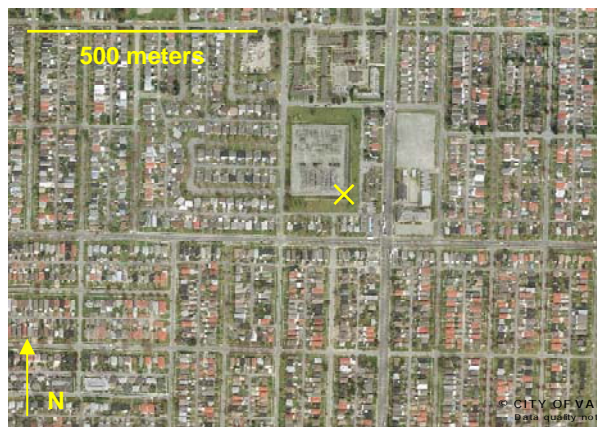
Figure 2: Airphoto of the suburban region. Tower location is marked with an X. (City of Vancouver, 2002)
