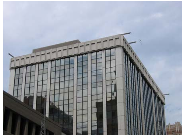
Figure 5. Photograph of the building located at the northeast corner of the Park Avenue urban canyon taken from the middle of the canyon at street level. A single 3D sonic anemometer is located on each of the visible corners of the building.
