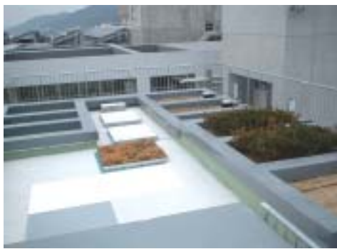
Picture 1 Experimental roof of Kobe University
