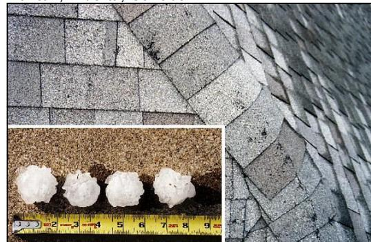
**Figure 6.** Hailstones to 2 in. (5.1 cm) in diameter and resulting roof damage in Flower Mound, Texas, in southern Denton County.
