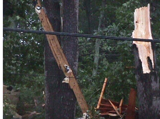
Figure 6. Part of the roof was nailed to a tree across the street. Photo by Glenn Field.
