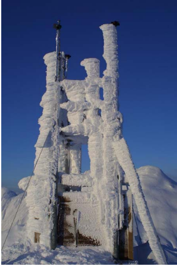
Figure 3: The Sheep Mountain anemometer tower shows buildup of rime ice. The anemometers are headed to protect from this vulnerability (courtesy Al Yates).
