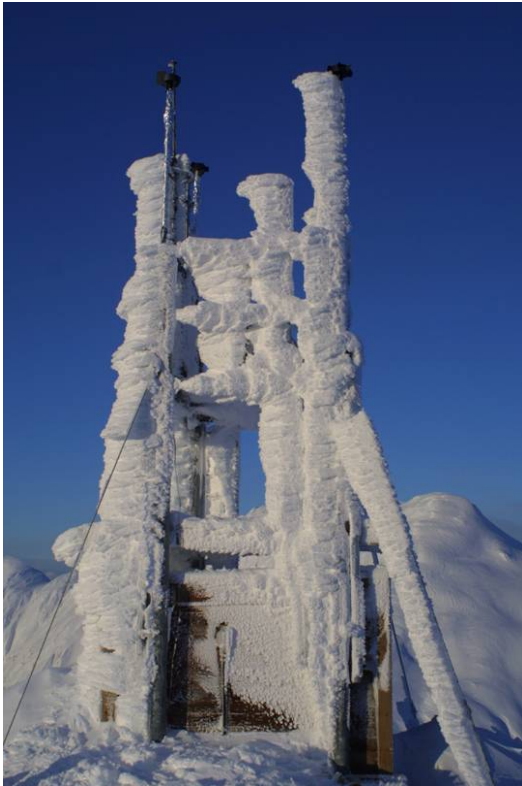
Figure 3. Sheep Mountain anemometer site after icing event
