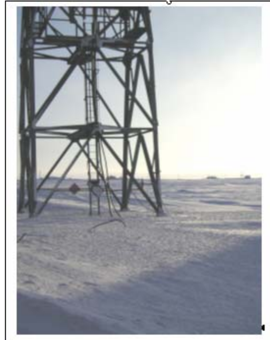
Figure 2. View along horizontal path from Barrow Alaska Dewline Towers to ARM 'Skydeck' building on the distant horizon.
