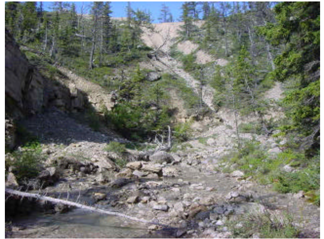
Figure 2: Colluvium washout from exposed Valley Walls into Milky Stream
