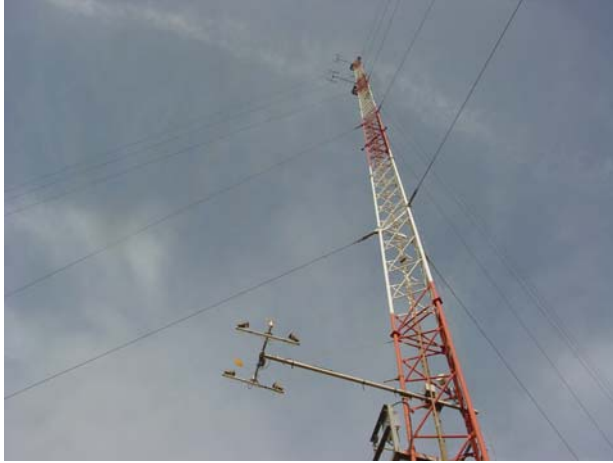
Figure 3. A three level meteorological tower similar to one at Dresden and LaSalle Nuclear power station.
