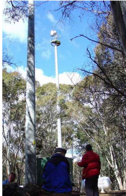
Figure 4. Elevated ground generator pair.
