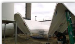
Radar wind profiler installation.
